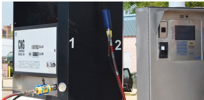
Hose Module installed on a natural gas pump; Ward Fuel Control Terminal
